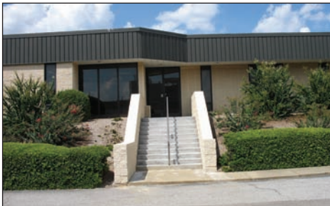
Olive Branch, Mississippi, USA Manufacturing and Distribution
