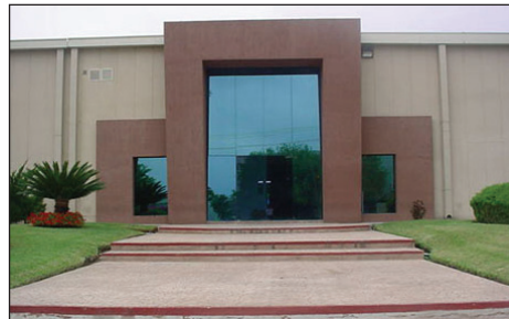
Monterrey, Mexico Manufacturing and Distribution
