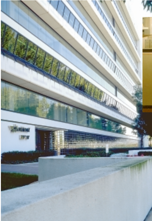
High windows above the light shelves allow deep daylight penetration.
